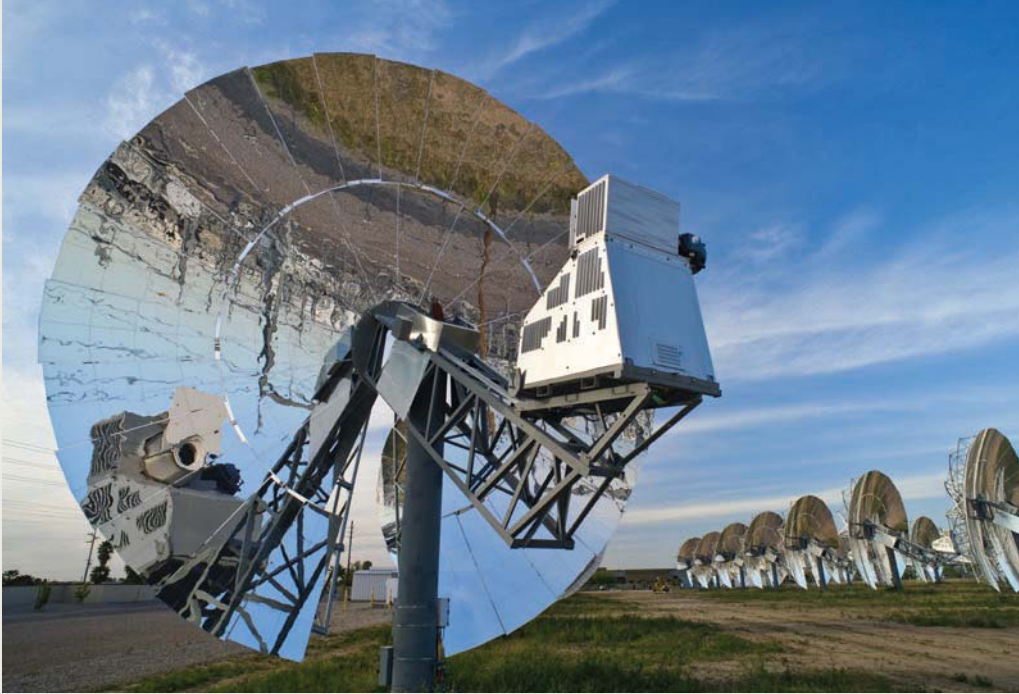
This giant mirror focuses sunlight onto material in the box.
